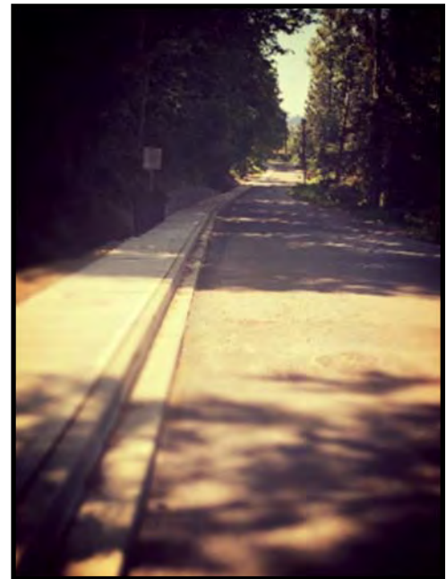
Callow Road—Sidewalk Complete—May 2018
