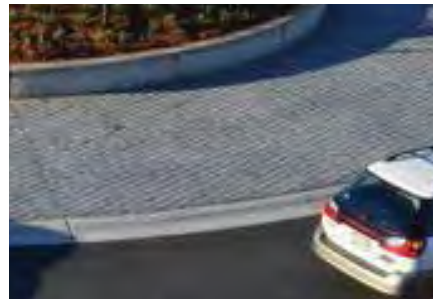
STAMPED MODULAR STONE CONCRETE IN ROUNDABOUT APRON
