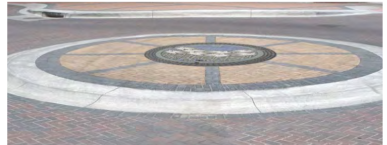
MOUNTABLE VEHICLE GRADE PAVERS (APPROX. 6"X6" CREAM/GRAY COLOR TONES) SET IN GEOMETRIC PATTERN WITH CENTER ART MEDALLION
