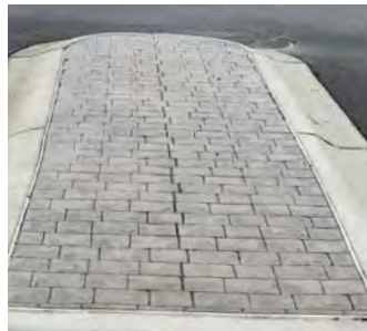
STAMPED MODULAR STONE CONCRETE IN MEDIAN ISLANDS
