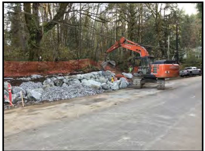
South Lake Stevens Road—Retaining Wall Construction
