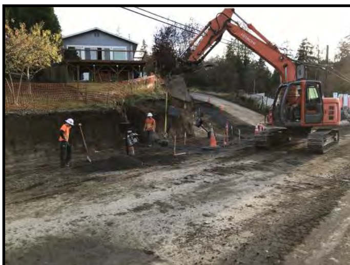
South Lake Stevens Road—Retaining Wall Excavation
