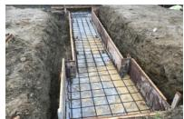
A new decant facility is under construction; a joint effort with the Sewer District supporting 50% of the cost. It is designed to receive, process and dispose of stormwater and sewer contaminates. The foundation has been poured and a new steel building on its way.
