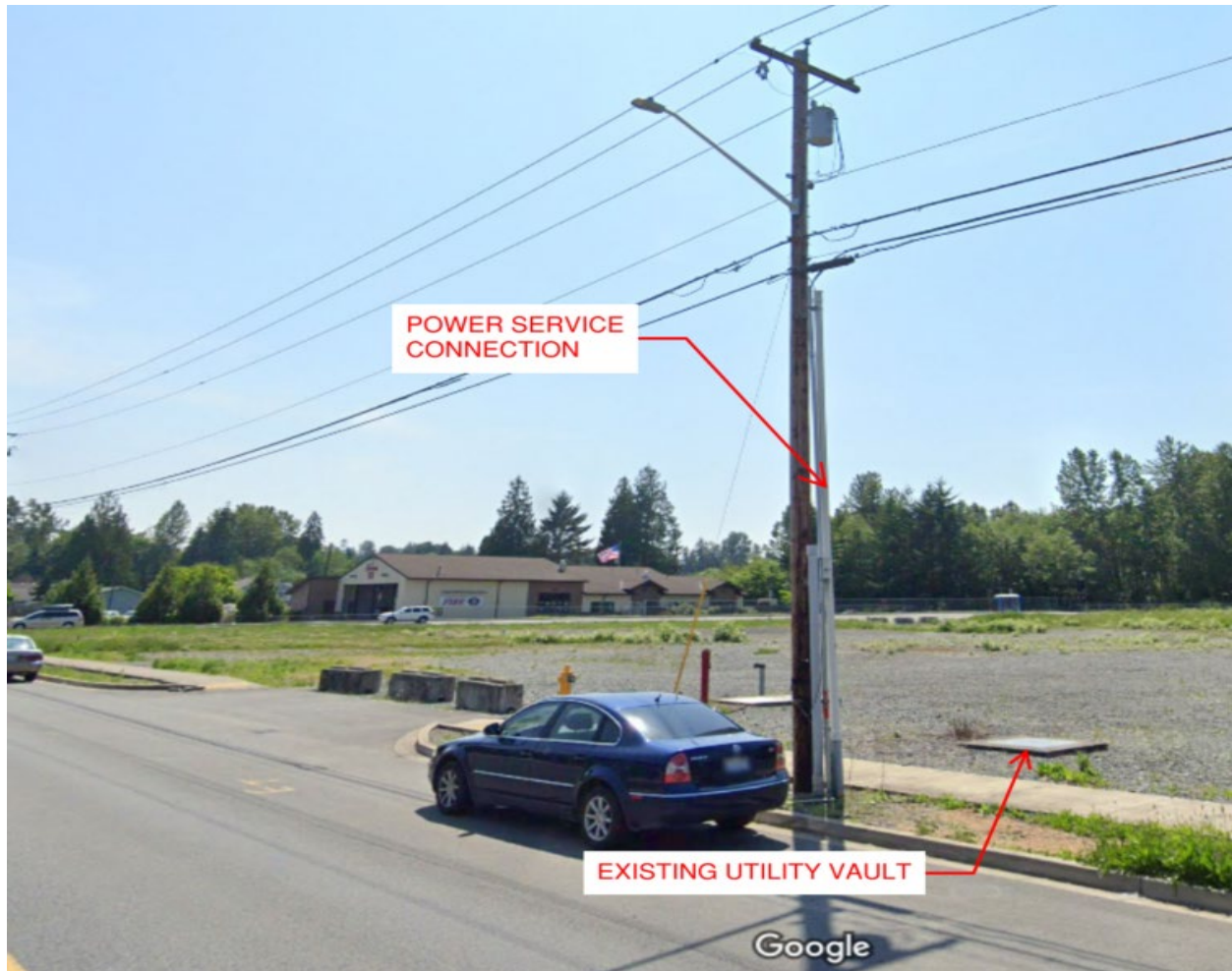
Figure 3. Google Street View Image of Site Power Service Connection.
