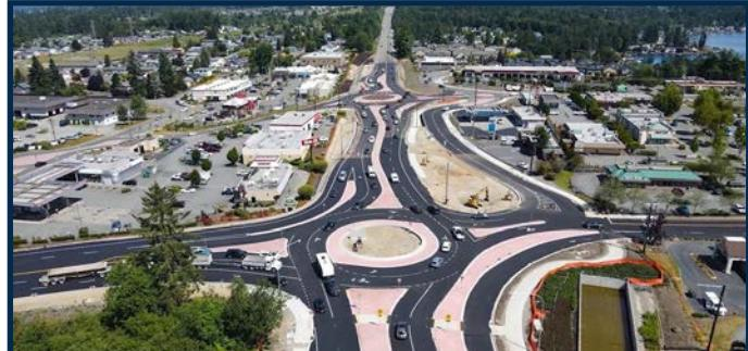
Over the past six years, WSDOT has worked on improving SR 9 and SR 204 by adding four roundabouts and widening SR 9 to four lanes. These improvements help manage congestion, improve mobility, and provide better access to area businesses. The city would like to thank WSDOT for all their hard work to make Lake Stevens a safe place to live and travel.
