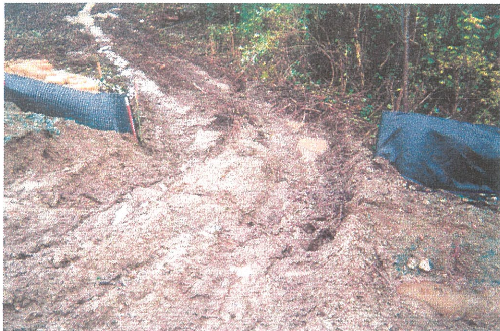
Figure 2-5 Breached Silt Fence Allowing Water and Sediment to Move Offsite
