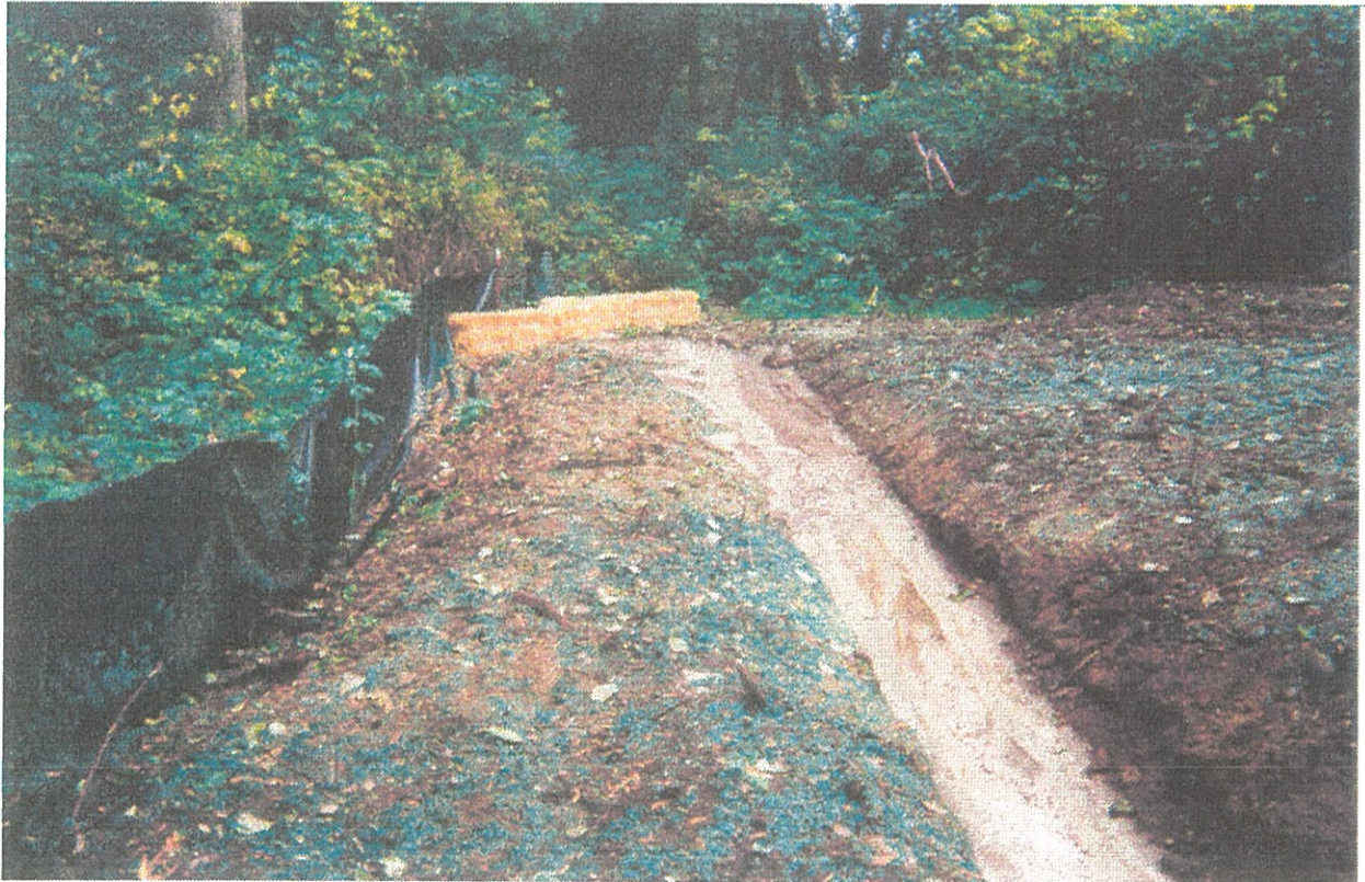
Figure 2-6 Storm Water and Sediment Moving Offsite
