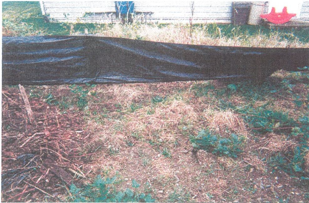
Figure 2-4 Silt Fence Installed but Not Keyed Into the Ground
