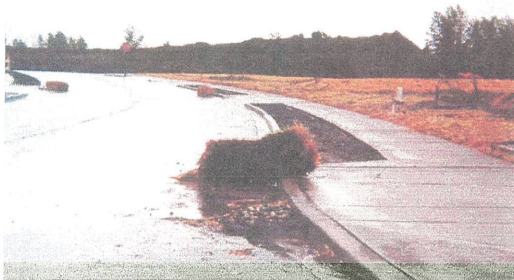
Figure 2-3 Ineffective Hay Bale Installation
