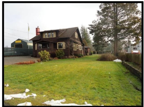
1. View of the subject property from 123 rd Drive NE, facing northeast.
