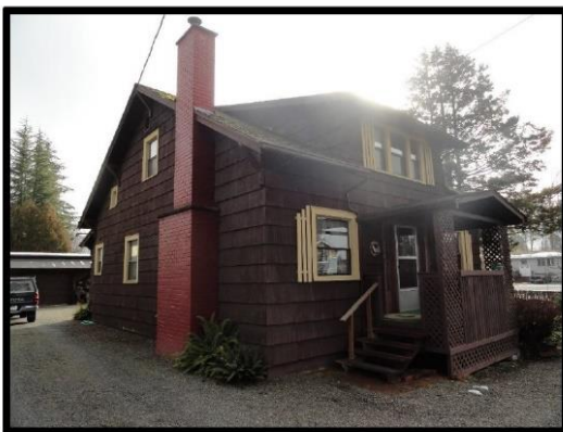
3. Front view of the single-family home, facing southeast.
